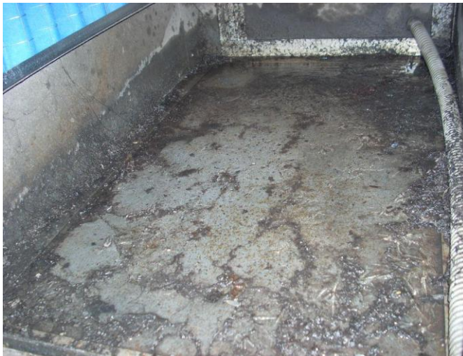
Ex. CONTAMINATED AHU
