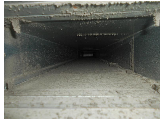
Ex. CONTAMINATED DUCT
